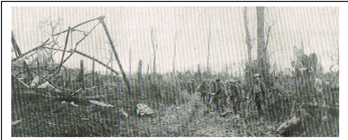
(Right: Pioneer troops building a road in newly-won territory – from Le Miroir)
