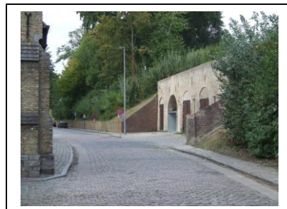
(Right: The entrance to 'A' Company's quarters – obviously renovated since that time - in the ramparts of the city of Ypres when it was posted there in 1916 – photograph from 2010 )
