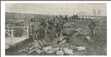
(Right above: Canadian personnel and German prisoners undertake the evacuation of the wounded from Vimy Ridge on a light railway which is still in the process of being constructed. – from Illustration )
