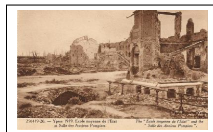
(Right: By 1918 Ypres was looking like this; some of these broken buildings had been a school which had served as a shelter for troops in the earlier days of the conflict. – from a vintage post-card)
