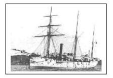
(Right above: The Redbreast-Class gunboat, HMS 'Sparrow', armed with six four-inch guns, was a sister-ship of 'Magpie'. – the photograph is from Wikipedia)
